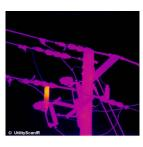
Properly functioning lightning arrestors should be uniform in temperature and close to ambient air temperature if they have not undergone recent solar loading. Individual arrestors should not have any pronounced hot spots across them. Working early in the morning, on cloudy days, or at night will help to eliminate solar loading which can hide defective arrestors. When performing your inspection, don't forget to check grounding connections for hot spots as well.
